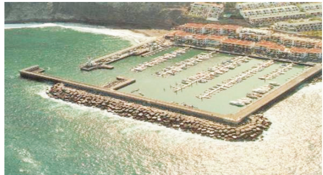
View of outer wall of a port structure
